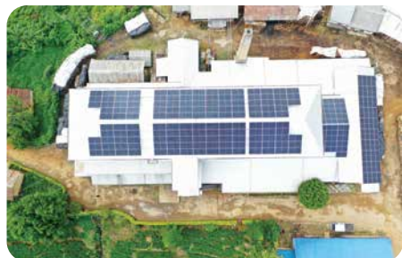
Factory rooftop solar - Bearwell Estate
